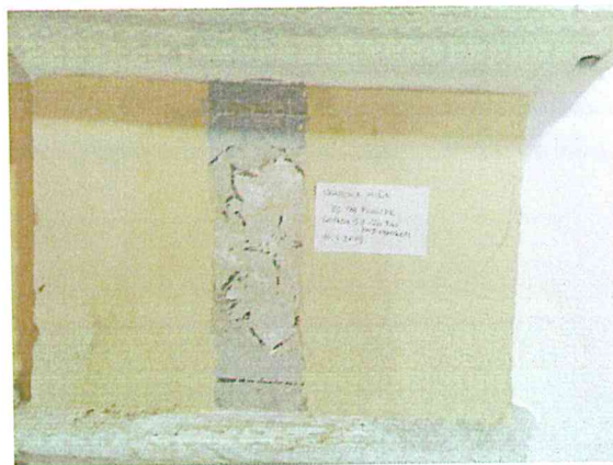
Foto 38: Sonda 31, pod obokom, pilaster
